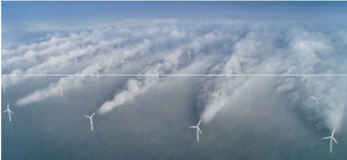
Plate 17: Illustration of the wind farm wake effect.
