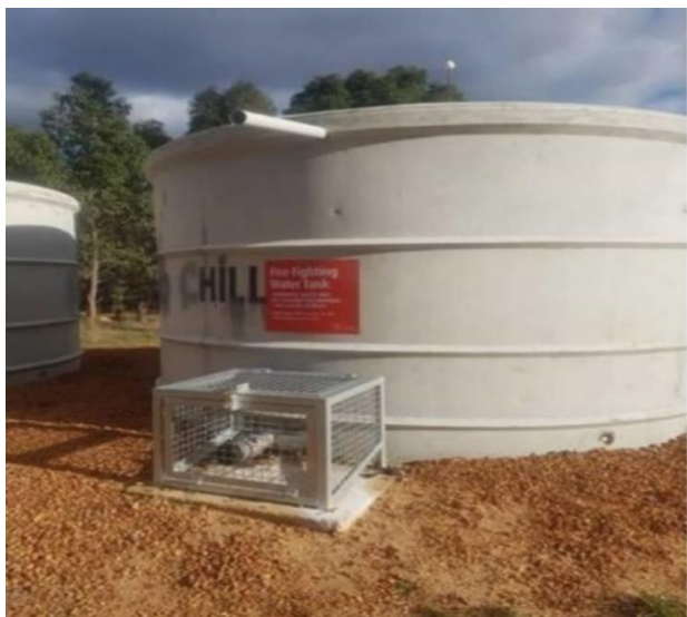
Strategic 47,000 Litre Concrete Tank & Protected Fittings
