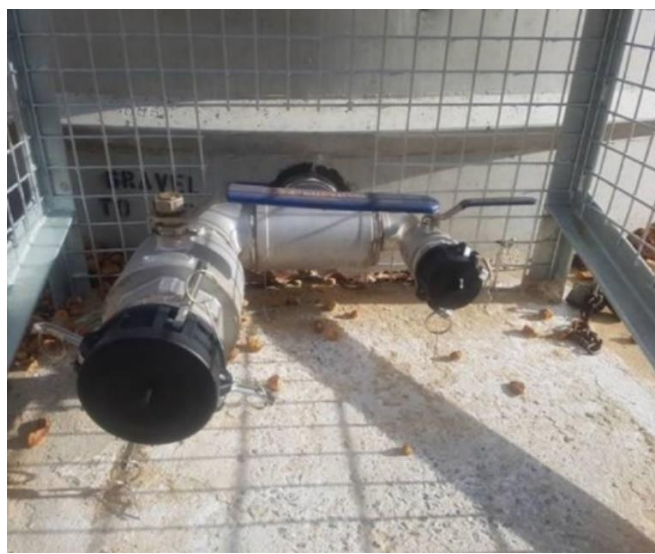
Strategic 47,000 Litre Concrete Tank & Protected Fittings
