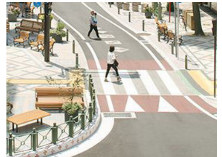
Raised pedestrian crossing
