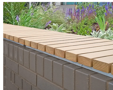
TIMBER SLATS - TO TOP OF WALL
