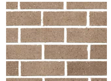
FACE BRICK WALLS
