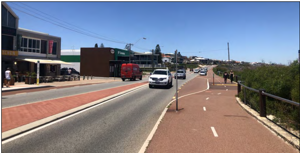
Photograph 2: Existing shared path as viewed from West Coast Drive, looking south.
