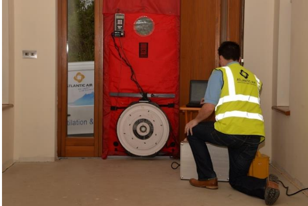
Figure 10.1 - Example of airtightness testing
