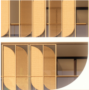
powdercoated and perforated aluminium sun-screening
