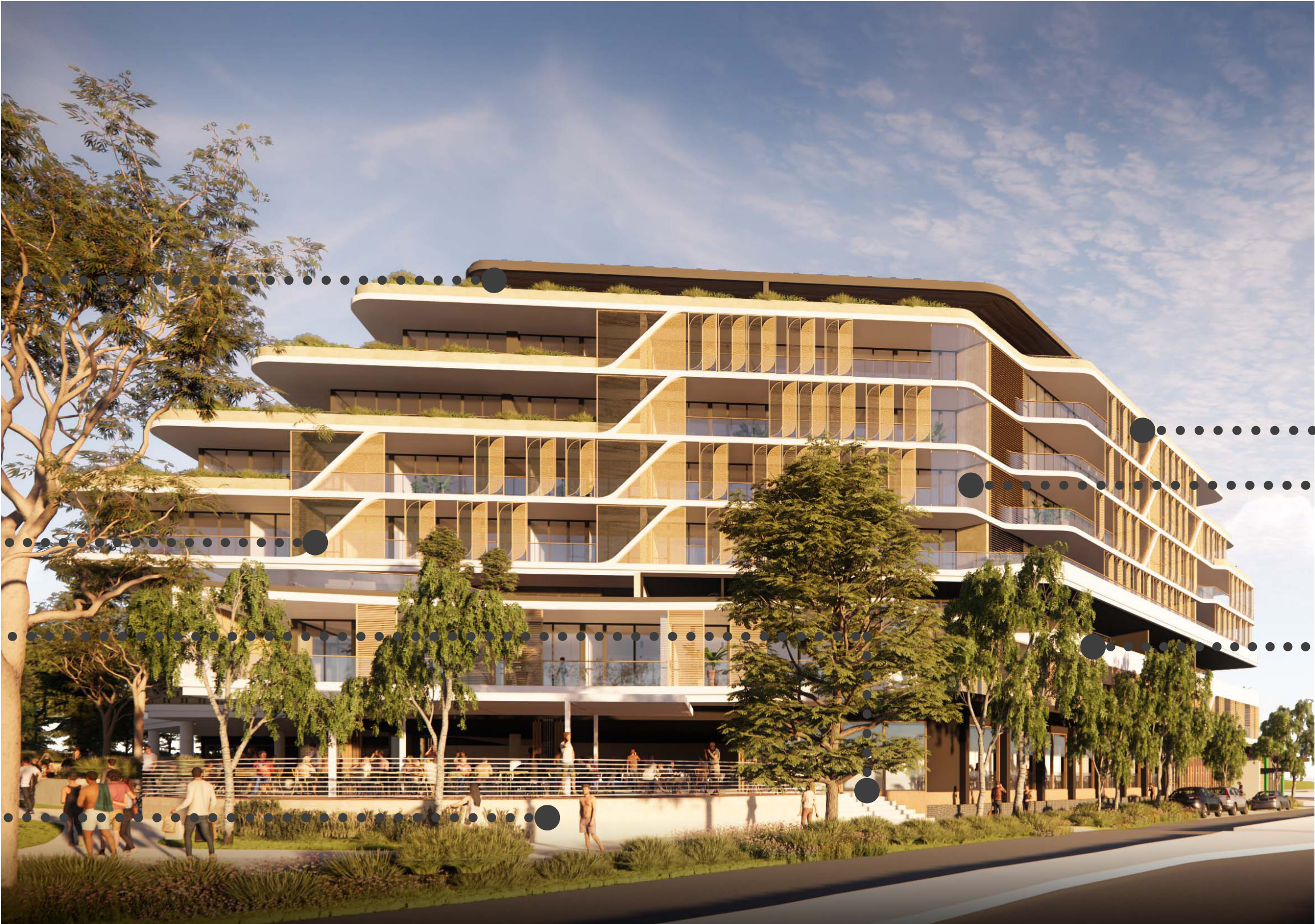
powdercoated and perforated aluminium sun-screening
