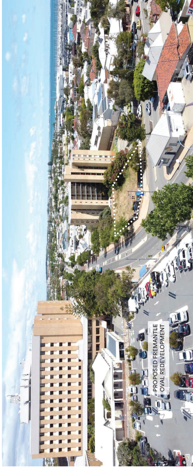
Aerial view of the Site looking South
