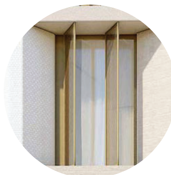
Aluminium sunshade screen detail (double screen)
