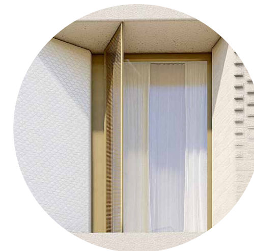
Aluminium sunshade screen detail (single screen)
