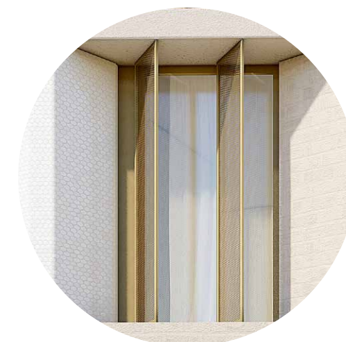
Aluminium sunshade screen detail (double screen)
