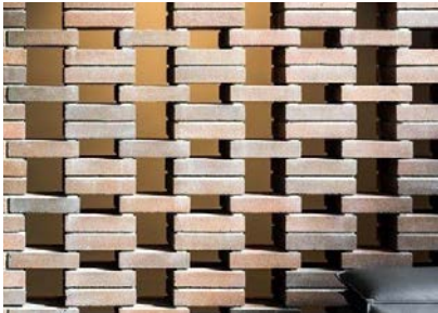
7. Lattice facebrick balustrade details to provide decoration and interest
