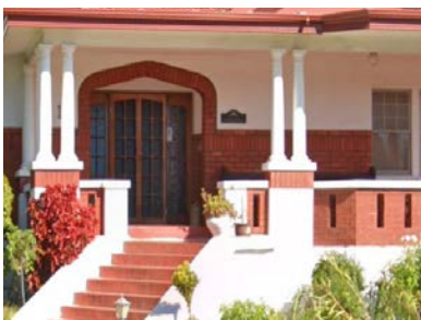
3. Decorative face brickwork used for building modulation and decoration.
