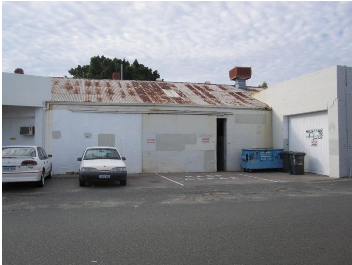
Figure 22 Rusted roofs and patched elevations and doors, 91 Canning Highway
