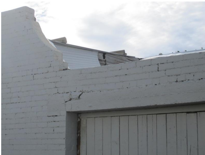
Figure 23 Failing brickwork and patched roofs, 91 Canning Highway
