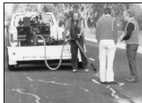
Filling and sanding cracks after routing
