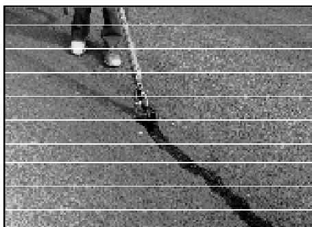
Crack filling with insulated hand lance
