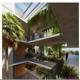
A key feature of the building is a landscaped east - west central axial void running the length of the building with suspended walkways and bridges connecting to the apartments at the various levels
